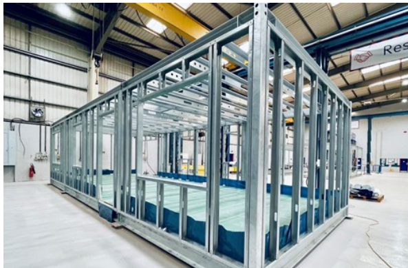
Figure 6 Skeletal Steel Frame (Totally Modular Limited)
