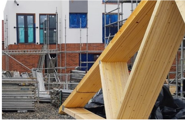
Figure 5 Prefabricated Roof Trusses for installation on site (Etopia)
